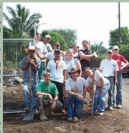
2003 YFC Project Serve Team in Guatemala, standing beside newly installed gate
